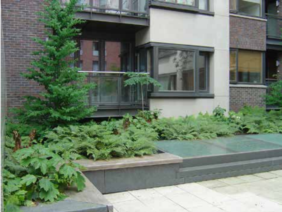
In situ block planters with stone and timber cladding (Ground floor open space and raised raingardens)
